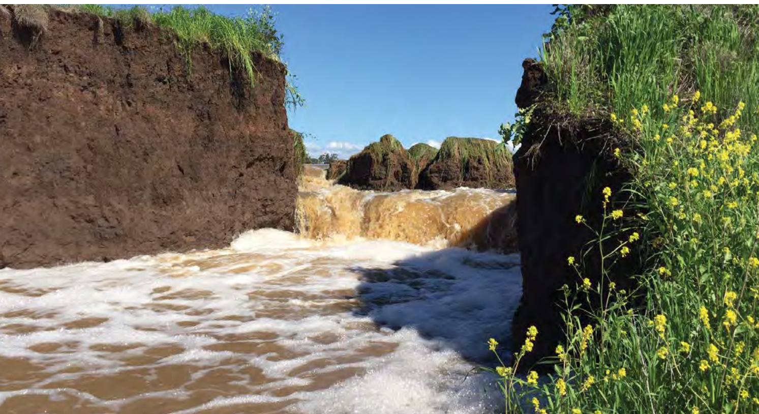
Failed storage. (PHOTO: STBIFM)
