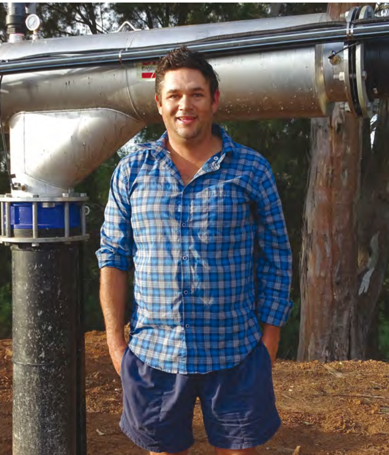
James Barlow in front of his new river pumping station.
